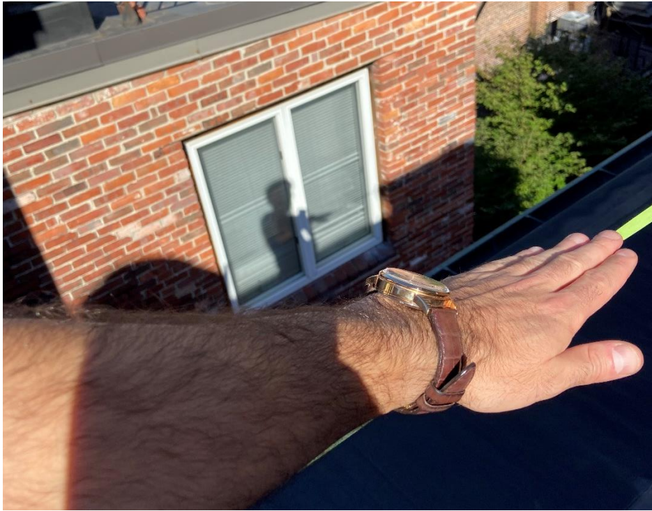
Figure 9: View of 58 Temple St. Window
