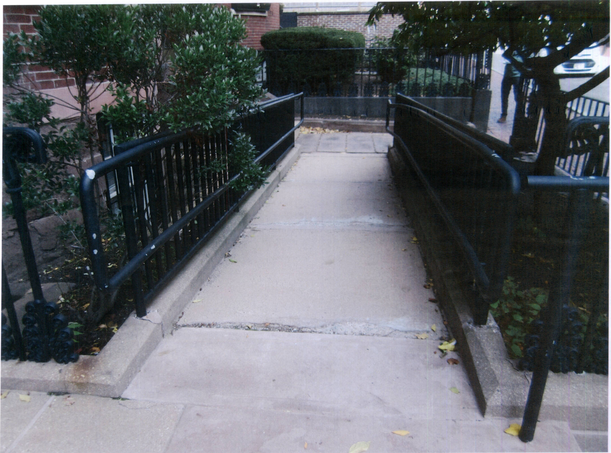
EXISTING RAMP @ #4 JOY FRONT
