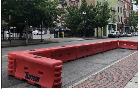
Water-filled jersey barriers To be filled with water by Licensee
